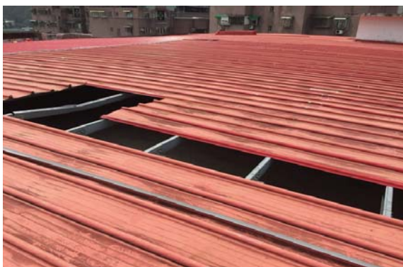
18 February 2017: Large Loot Storage roof prior to the repair
