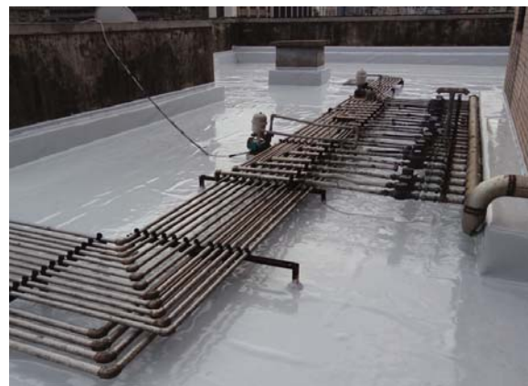
20 December 2015: existing roof waterproof layer after the repair
