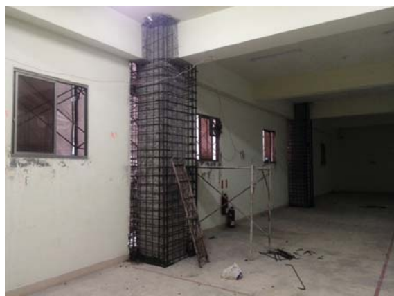
20 October 2017: during the loot storage's expansion column reinforcement
