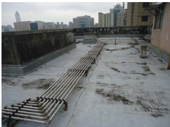
2 October 2015: existing roof waterproof layer prior to the repair
