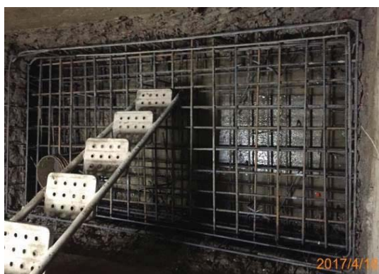
18 April 2017: adjust depth of the dumbwaiter manhole
