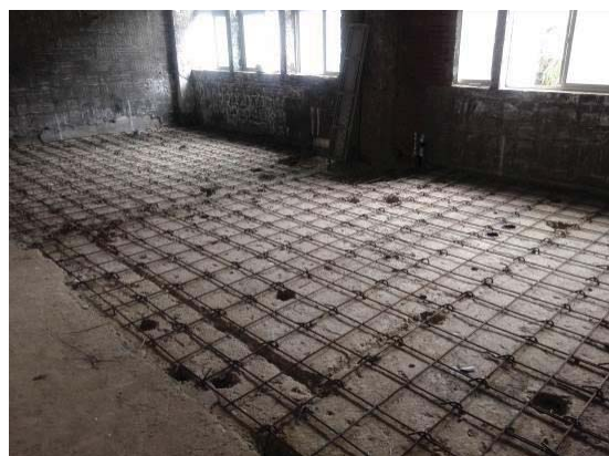
22 May 2017: floor slab reinforcement
