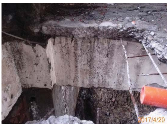
20 April 2017: floor slab used only single layer of No.2 reinforcement
