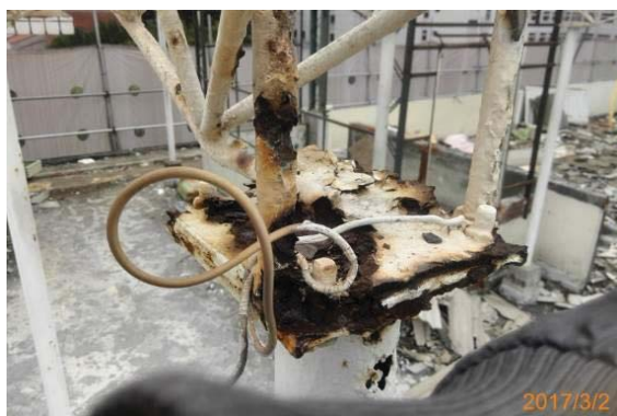
2 March 2017: rusted roof struss
