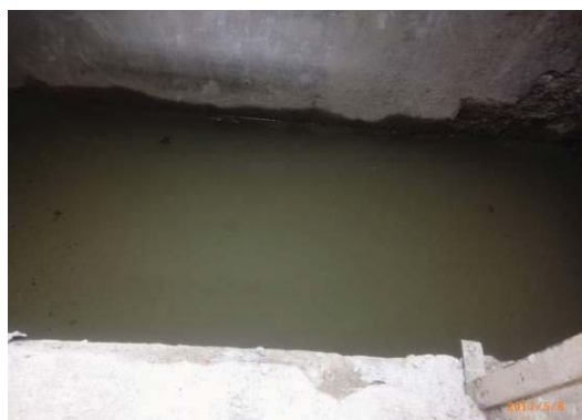
8 May 2017: dumbwaiter manhole water seepage
