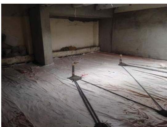
18 September 2017: drain water by crushed stone & non-woven fabric
