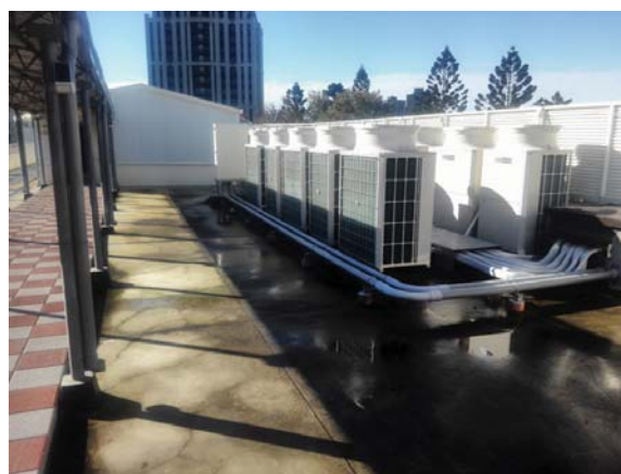
29 January 2018: 4/F, VRV air-conditioner compressor (outdoor)
