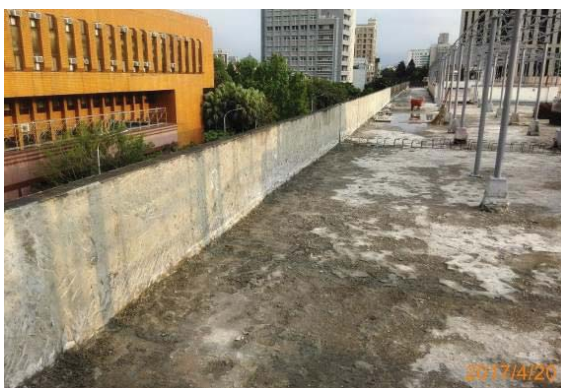
20 April 2017: construct waterproof slope
