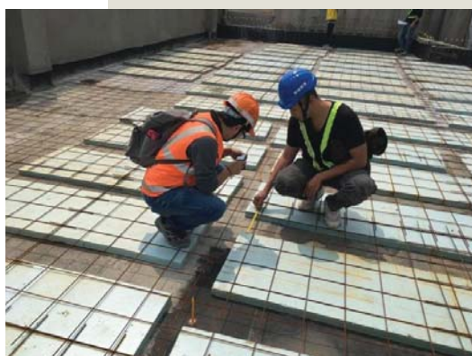
2019.03.27 The hot insulation and rebar nets check of roofs
