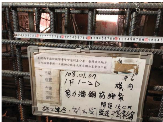
2019.01.07 The reinforcement examine of shear walls
