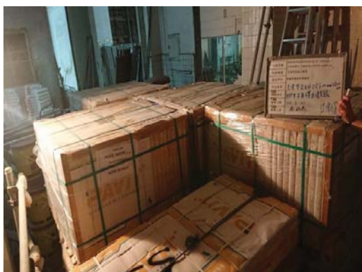
2019.03.21 The examine of polished quartz bricks in arrival
